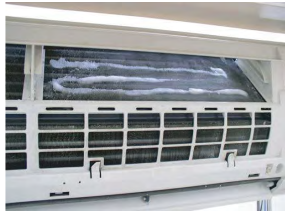
Step 3b: Allow the foam to penetrate for 30 minutes.
