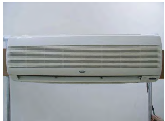
Step 4b: Switch on the Air-Conditioner to high modes set the temperature to about 24°C. Allow cleaning for 45 min - 1 hour
