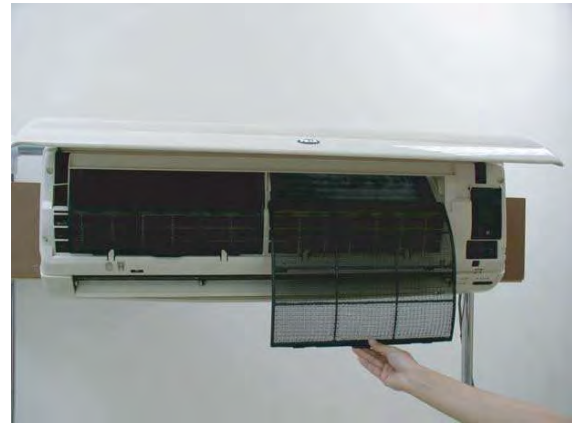
Step 2: Remove the filters for rinsing. Expose cooling fins and coils.
