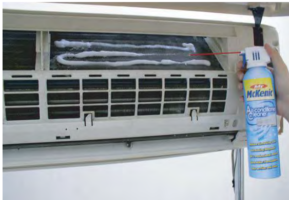
Step 3a: Shake can well before use. Spray approximately 10cm away in a horizontal motion from top to bottom. Do not overspray! Cover 30% of this only
